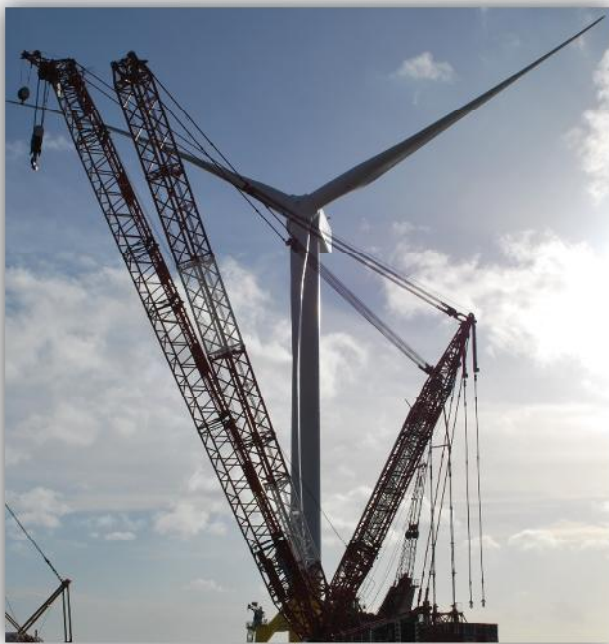
Construction of a Turbine
